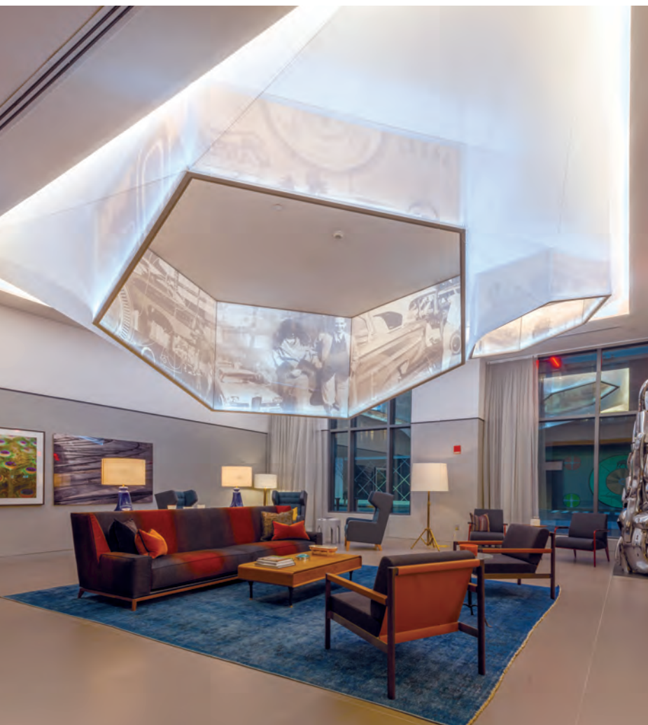
A stretched, translucent fabric ceiling at the Montaje Apartments, Somerville, Mass., combines dye-sub graphics and programmable lighting. The lighting structure is designed by Planeta Design Group and Transformit; fabrication and installation by Transformit. Photo: Transformit.
