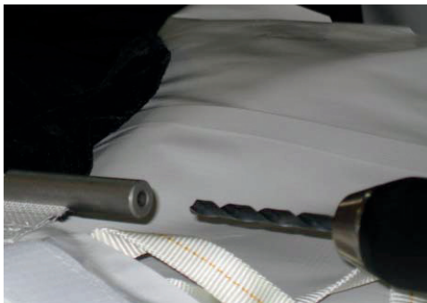
Drilling the Keder
